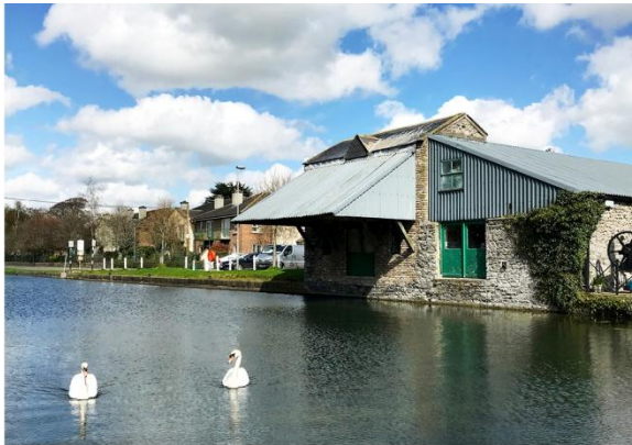
Figure 8.20 Harbour Basin and Former Warehouse
